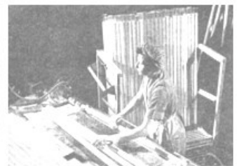
Cleaning Tube Ends, 1948 (1)
