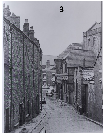
Some of the buildings have been demolished.
