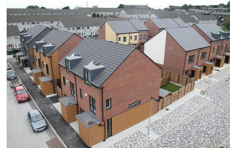
5. St Mary's new builds
