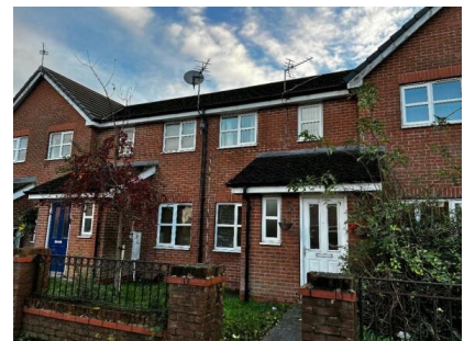
4. Limeside new builds
