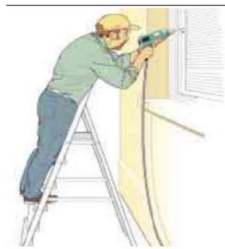
Correct – steps facing work activity
