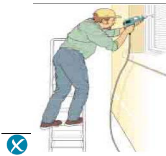
Incorrect – steps side on to work activity
